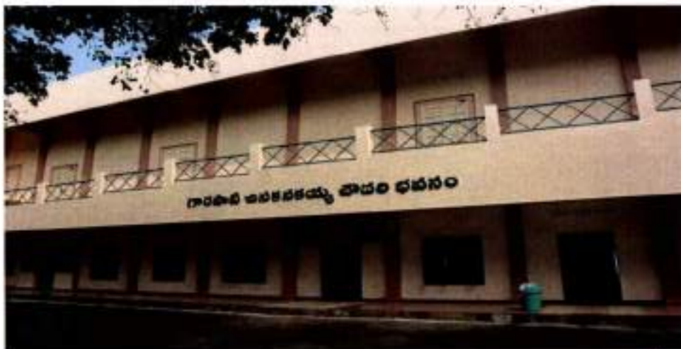
Photo.15 Canteen & AC Auditorium
