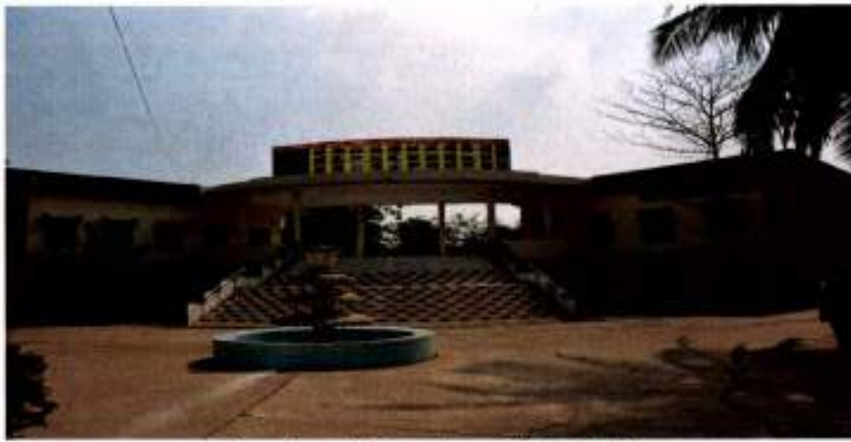
Photo.1 Administrative Office & Library
