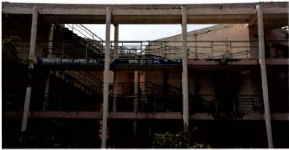
Photo.7 Mechanical Engg Block 3
